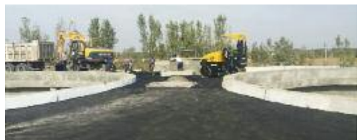
Rehabilitation of Primary Settling Tanks, Andijan, Uzbekistan
