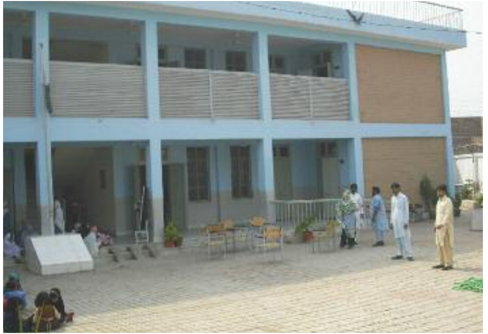
Girls' Primary School in Dag Bahsud, Nowshera District: Extension Building from 2016 with 8 Classrooms, Sanitary Facilities and School Yard Improvement
