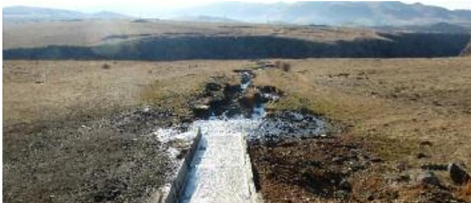
Outlet channel of right bank main irrigation canal and erosion problems due to uncompleted construction
